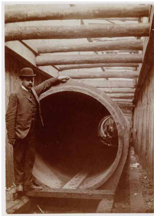
Sewer construction, Amsterdam, 1910–12. Copyright: Stadsarchief Amsterdam, CCo.
