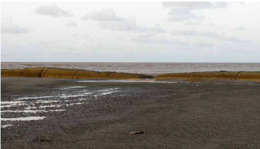
↑ Seaweed on the surface of a soft groyne.
