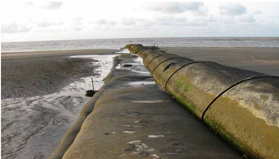
← Typical soft groyne in Guyana.
