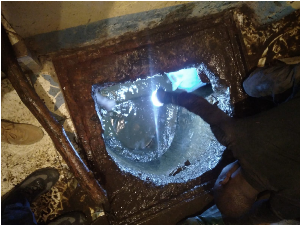
Biogas toilet tunnel cleaning at night. Photo: Mwangi Mwaura, February 2023.
