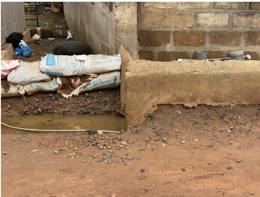
Sand and nylon bags used to construct flood barriers in the upmarket and upstream neighbourhood of East Legon, Accra. Photo: Afra Foli, 2020.
