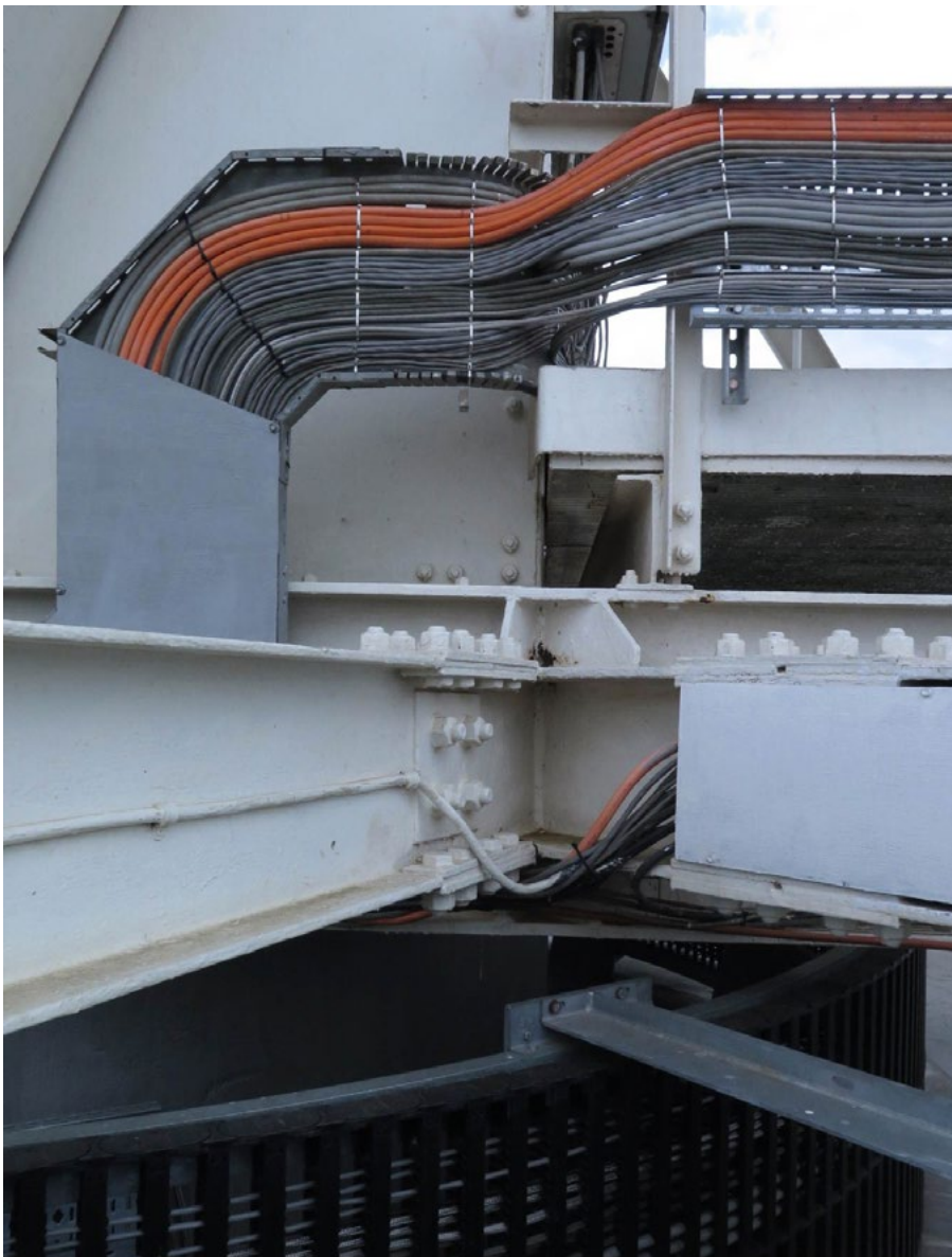
Cable wraps that transport data and power from the receiver to high-performance computers in the laboratory below. Photograph: Andrea Zimmermann, August 2019.
