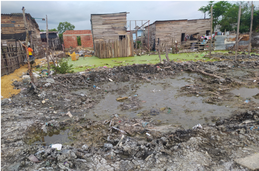
Bare ground in Playa Blanca. These houses are near one of the canals leading to the swamp. Photo: Maria Buelvas, 2021.
