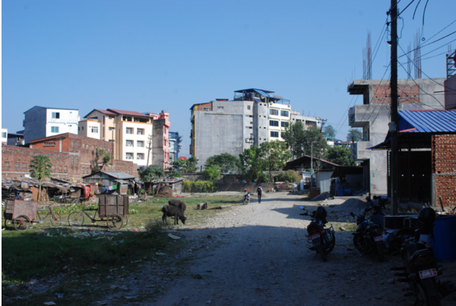
Gravel road after drainage has been installed, informal settlement on the left. Photo: Hanna Ruszczyk, 2017.
